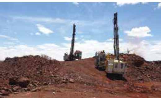
GD5000 drills are being used on the project.
